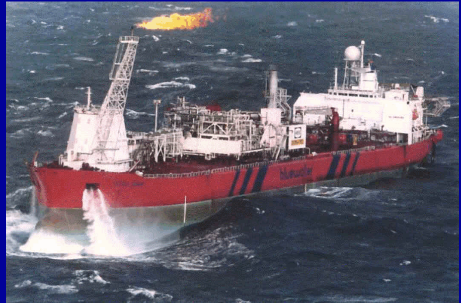
Photo courtesy of Bluewater Offshore
