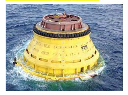
2 of 7 5/5/17, 12:00 PM Shell's Stones project features the largest disconnectable buoy built for the oil and gas industry to date. The buoy was designed for use with steel lazy-wave risers. Photo from SBM Offshore.
