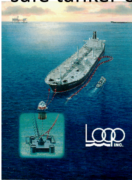
Offloading to CALM Buoy offshore
