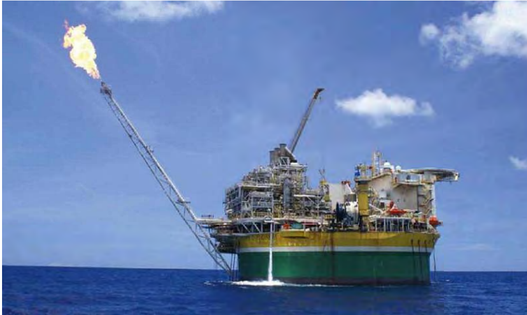
Sevan Piranema , credited as being the first round-hulled FPSO; her 64.3m diameter is not so far from the Ark's diameter of 63.2m
