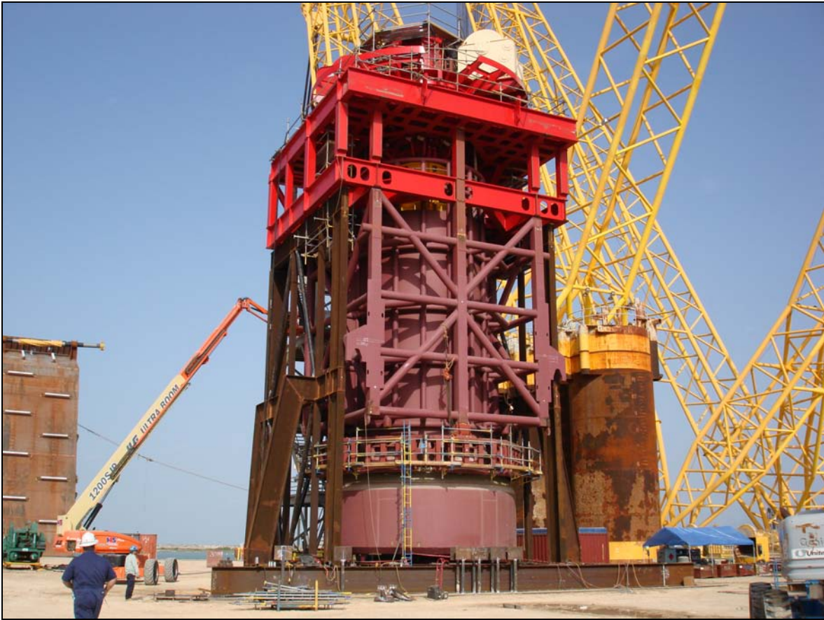
Figure 21. Disconnectable transfer system to attach the Helix Producer 1 to the subsea wells in the Phoenix Field. (Photo courtesy of Helix Energy Solutions.)
