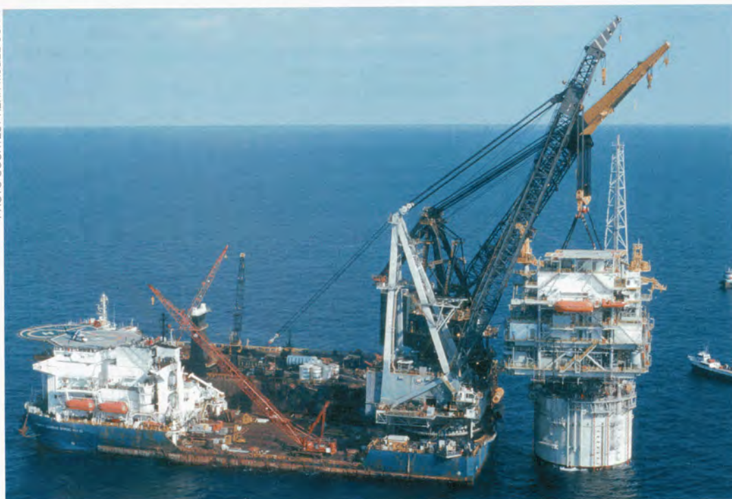
Deepwater infrastructure is massive. Here, two McDermott International crane barges lashed together to lift the 5,300-ton topsides of Kerr-McGee’s truss spar onto the hull at Nansen Field in the East Breaks area.
